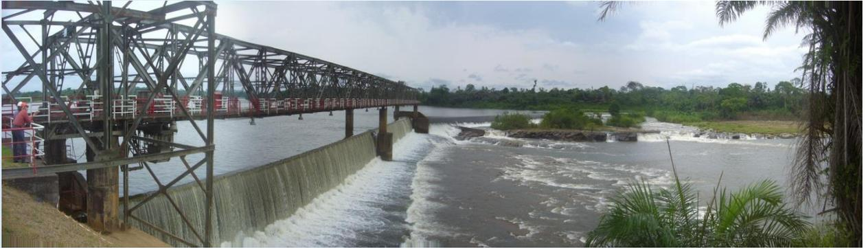
Situation in March 2008 during ending of flooding period. The old spillway system was built in the 50s and is no longer safe. In consequence the whole EDEA Hydropower plant and with it the Alucam aluminium factory in Edea as well as the south of Cameroon private consumption is in big danger of huge energy losses. The new modern spillway system will be built 6 m downstream of the old dam axis.
